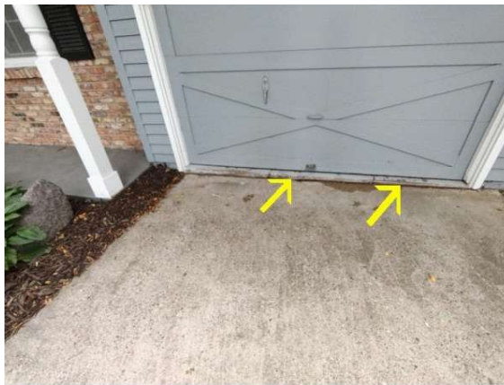
deteriorated block below slab
