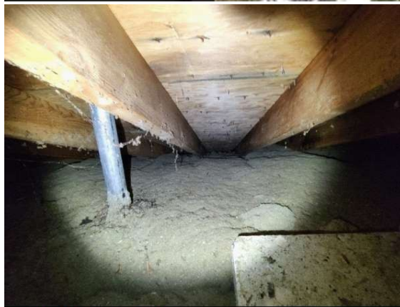
no baffles installed
