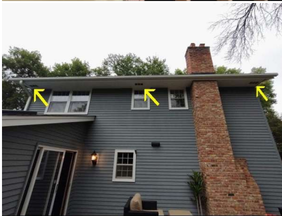
inadequate number of vents
