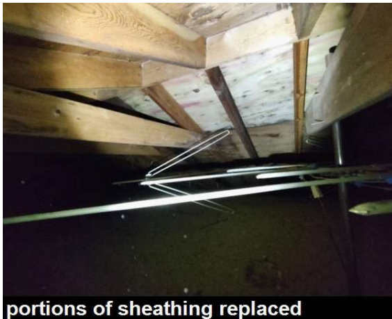
delaminated sheathing
