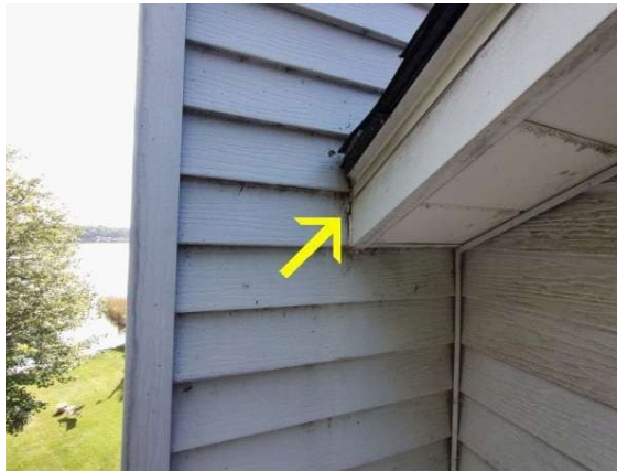
water has drained through gap
