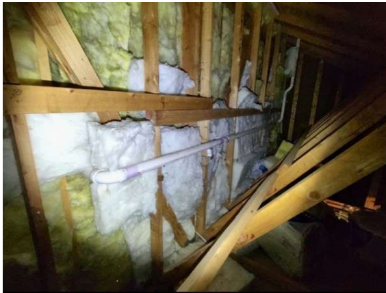
exposed vent plumbing
