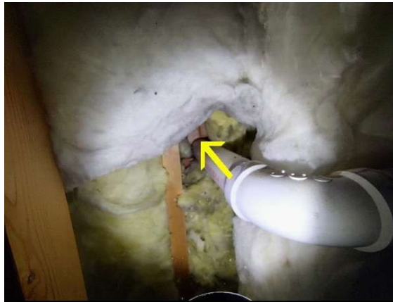
gaps where pipes penetrate
