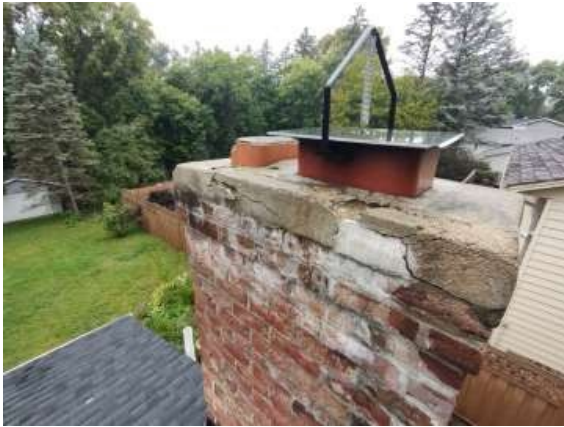
damper damaged - does not operate
