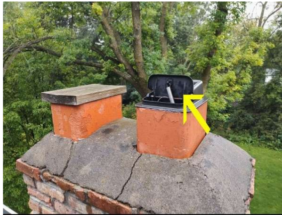
damper damaged - does not operate
